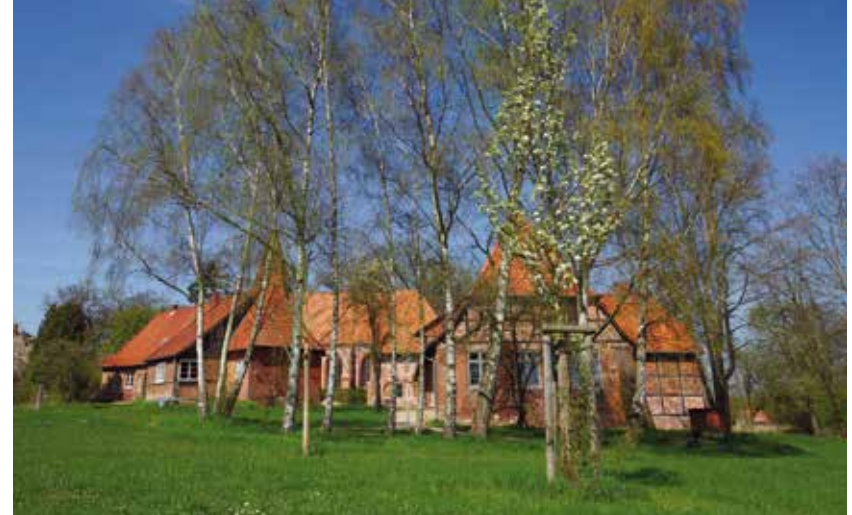
St. Nikolaihof, Bardowick
